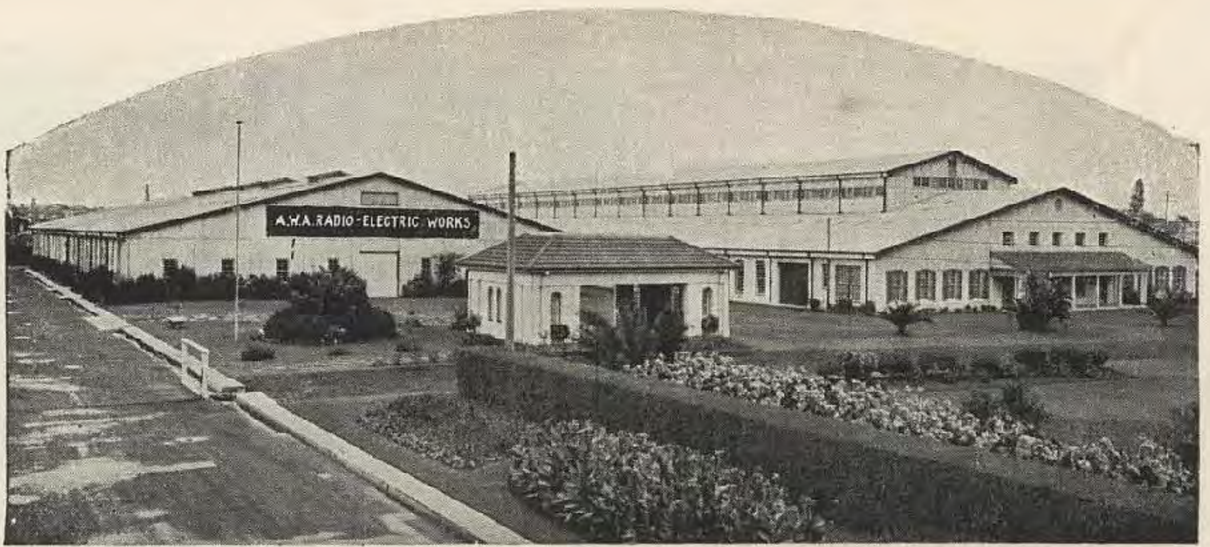
AN AUSTRALIAN FACTORY IN AN AUSTRALIAN GARDEN
